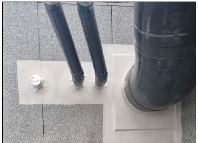
Liquid detailing around penetrations
