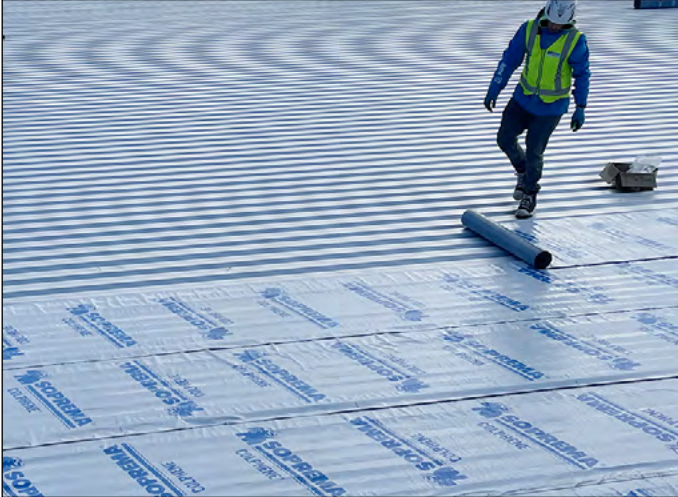
Installation of the vapour barrier over steel tray
