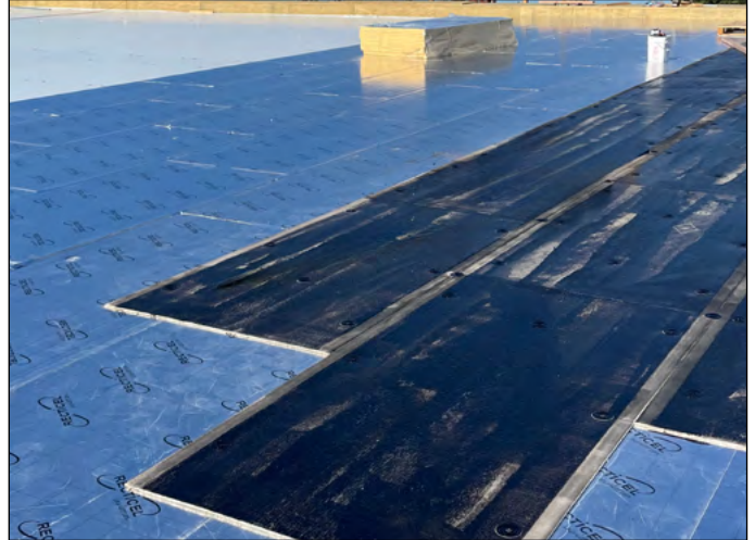
PIR insulation with mechanically fastened roof board over the top
