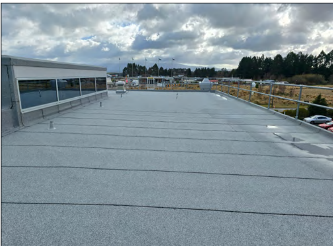
Cap sheet applied
