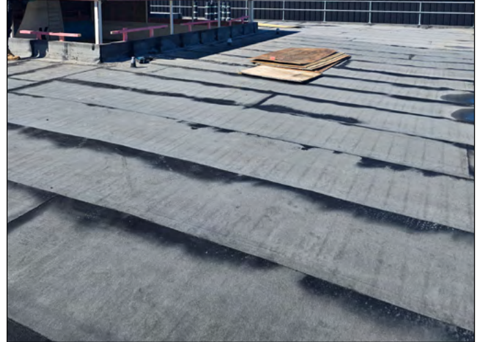
Base sheet laid
