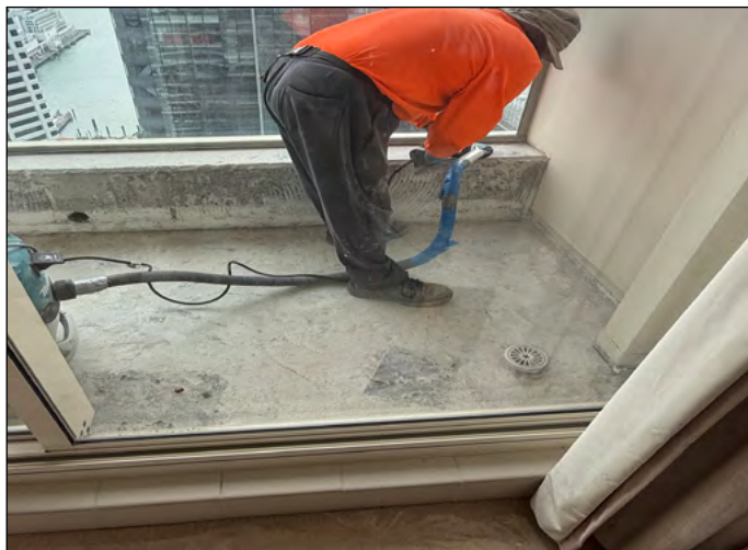
Removal of the existing screed and membrane
