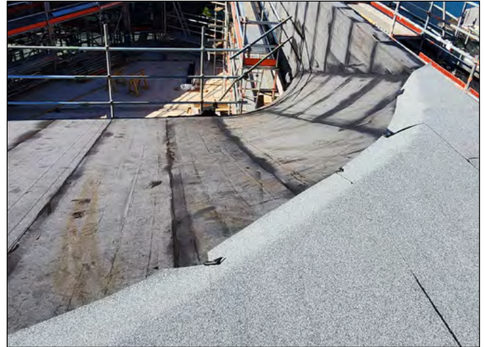
Base sheet laid, cap sheet installation
