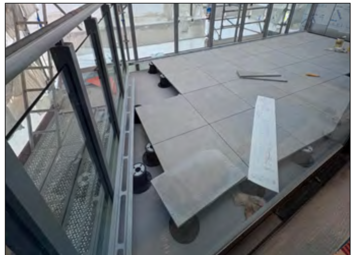
Ready for cut tile installation
