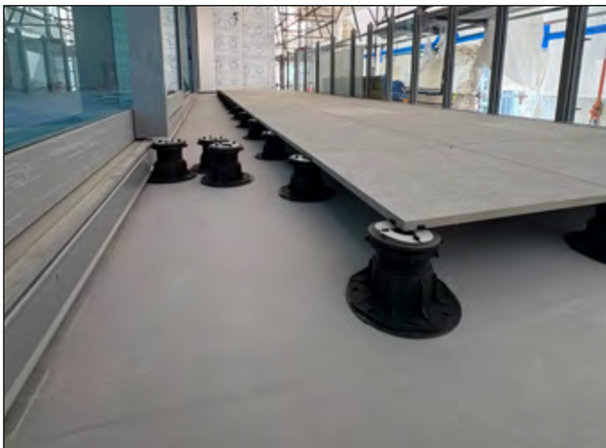
Full tiles installed and levelled
