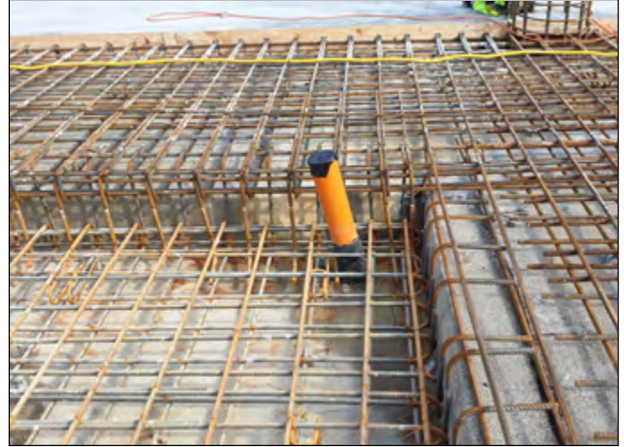
Steel reinforcement over completed tanking
