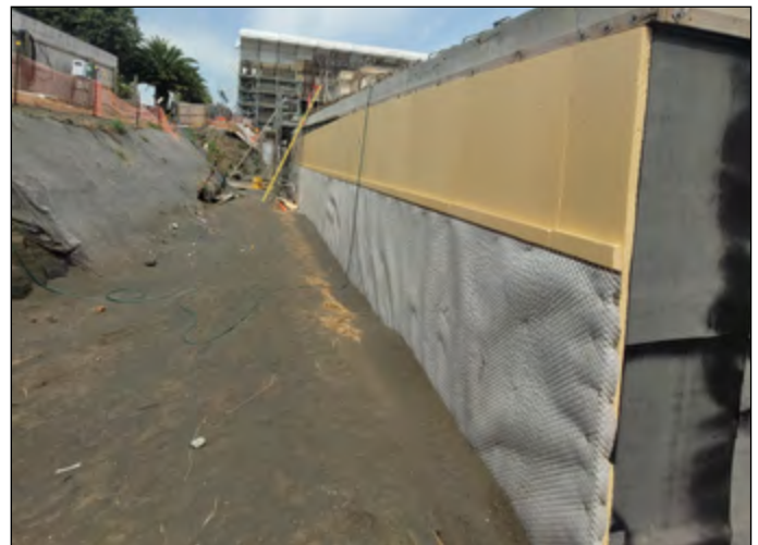
Insulation and drainage layer installed
