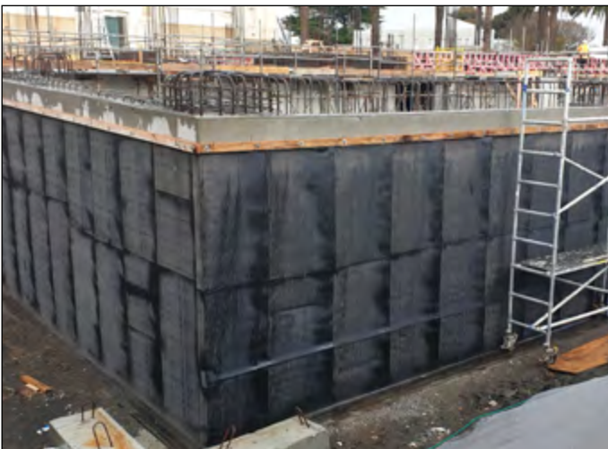
Tanking membrane installation
