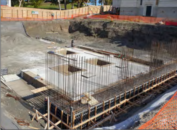
Column and footing tanking
