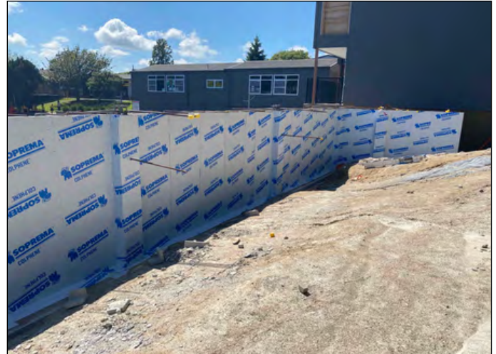
Installation of COLPHENE 3000 below ground waterproofing membrane
