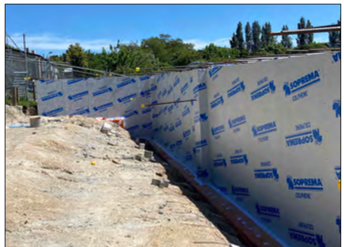
Connection of COLPHENE 3000 waterproofing membrane to DPM
