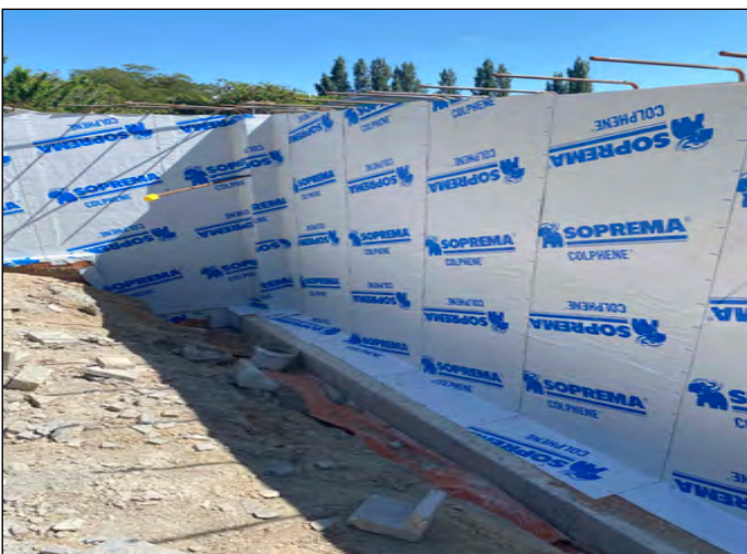
Completed wall waterproofing
