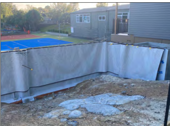
Installation of Equus drainage, filter and protection layer
