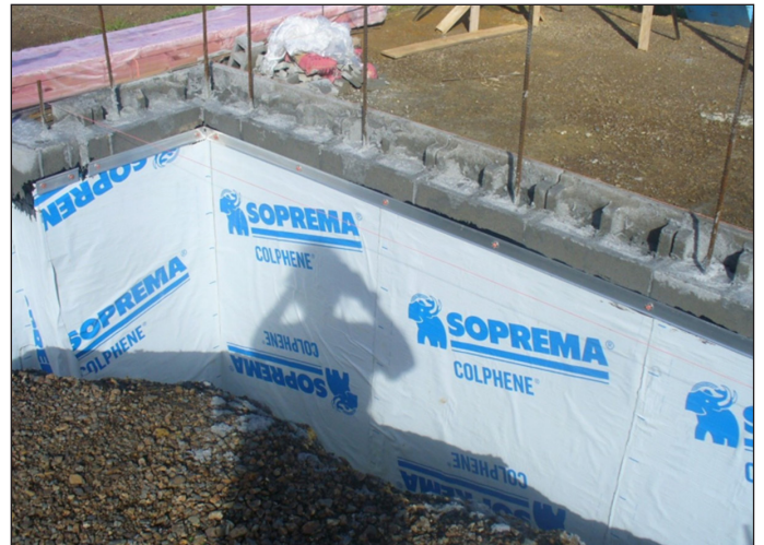
COLPHENE 3000 waterproofing membrane to wall
