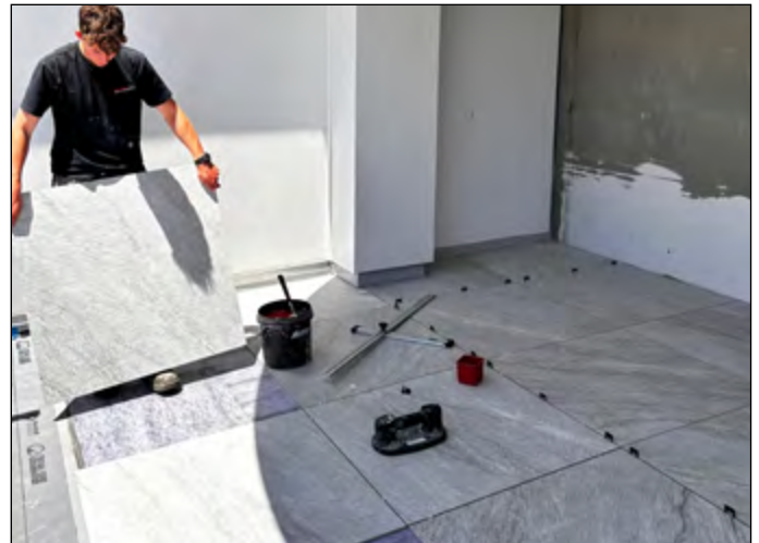
Tiles installed using Unifix-S3 tile adhesive and Cristallfuge Plus tile grout
