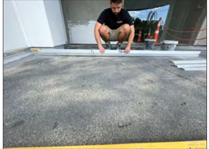
Tiler preparing for tile installation over Matacryn liquid applied membrane
