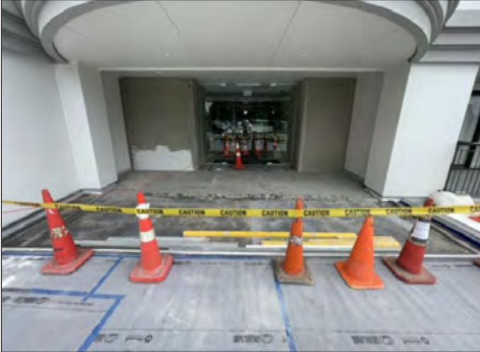
Matacryn liquid applied membrane installed on suspended concrete substrate
