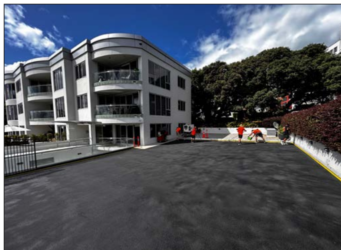
Second and final application of Matacryl STC (Clear) Topcoat
