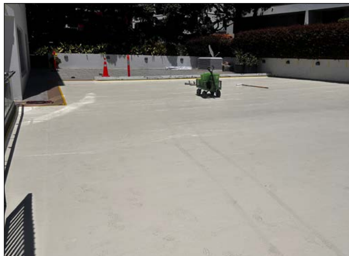
Matacryl waterproofing layer applied
