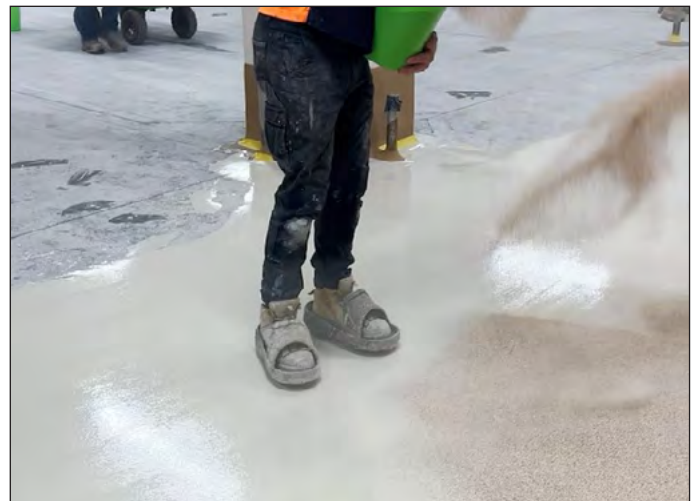
Broadcasting the aggregate onto the body coat
