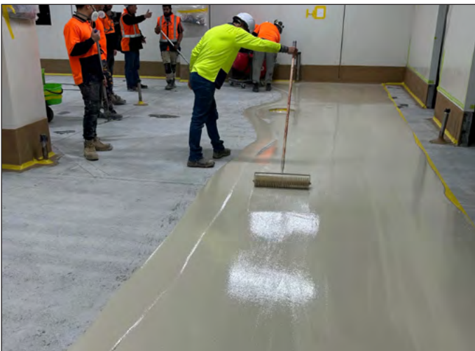
First layer of body coat
