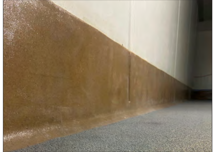
Epoxy cove installation
