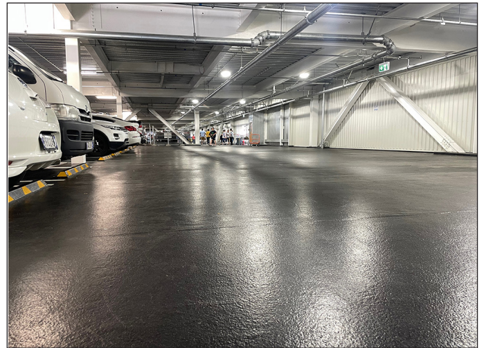
First and second topcoats of Matacryn STC (tinted black) applied
