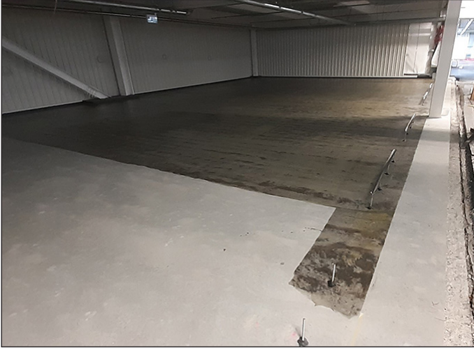
Substrate prepared and primed
