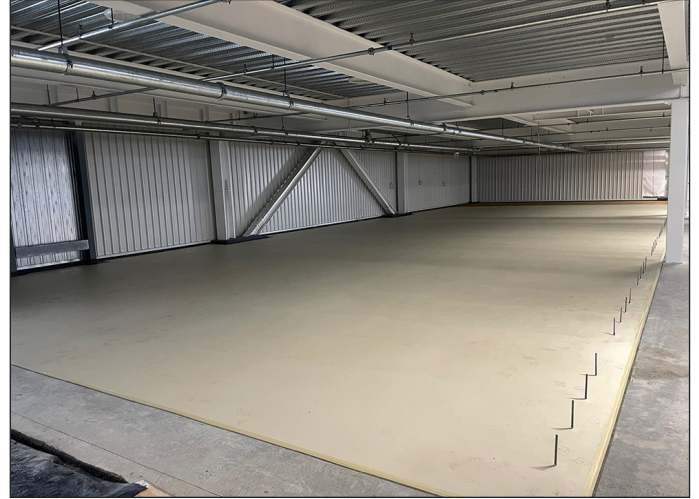
Matacryn Manual membrane layer laid
