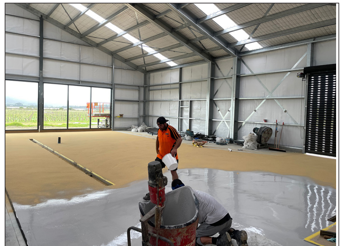
Broadcasting the aggregate onto the body coat
