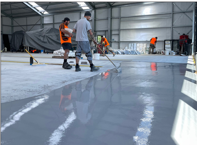
First layer of body coat
