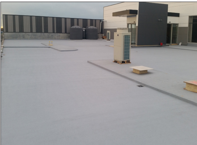
Application of Matacryn carpark membrane
