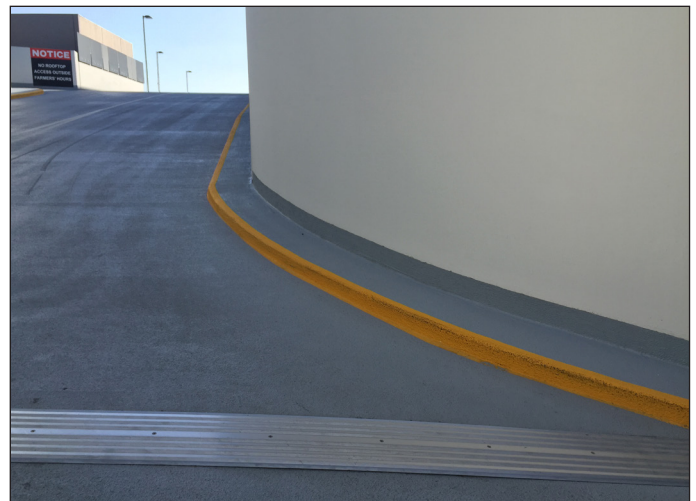
Completed Matacryn carpark membrane on ramp
