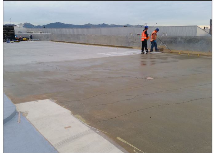
Primer application to concrete substrate
