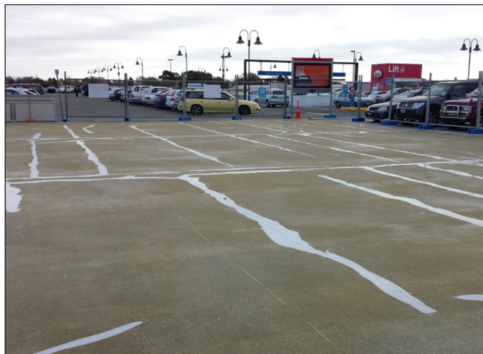
Crack repair to existing substrate
