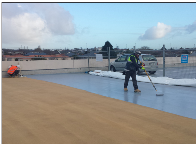
Application of Matacryl carpark membrane
