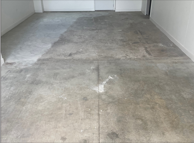
Existing garage floor
