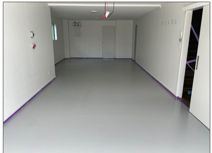
Epistix Rapid Topcoat applied over Epistix primer
