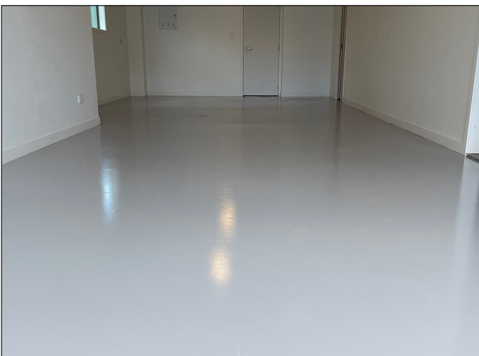
Additional coat of Epistix Rapid Topcoat applied to complete the project
