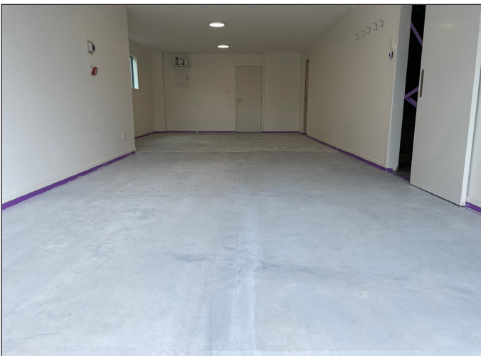
Epistix primer applied to existing concrete
