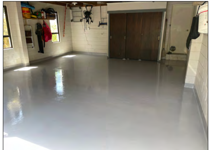
Epistix Rapid 3x coat system applied to concrete
