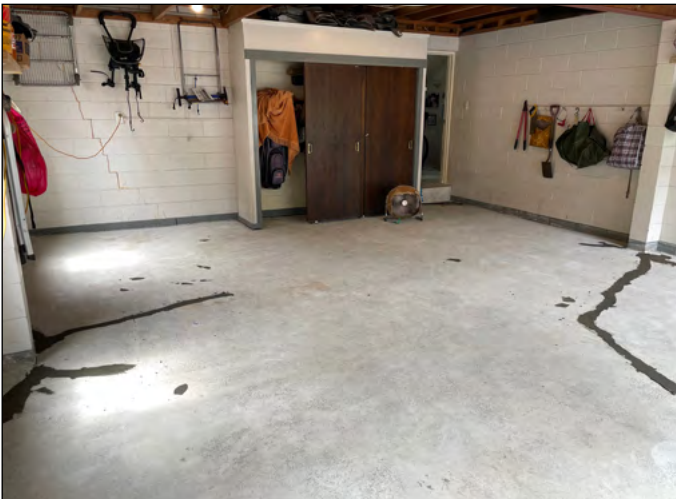
Surface preparation – existing coatings removed by diamond grinding
