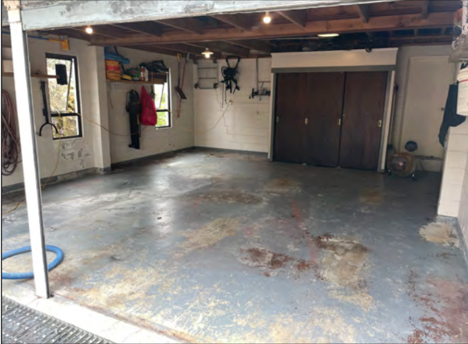
Existing garage floor
