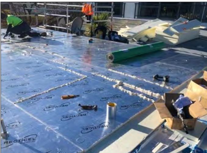
PIR insulation, mechanically fastened to provide additional thermal benefits
