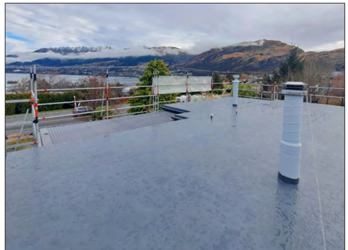
Installation of Flagon TPO waterproofing
