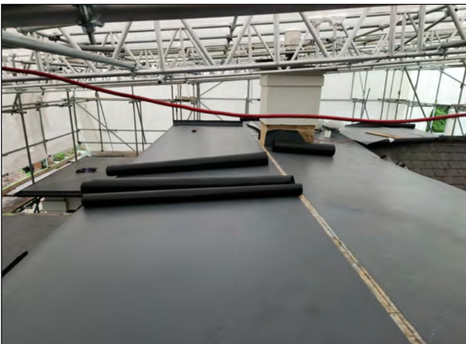
FLAGON TPO installation
