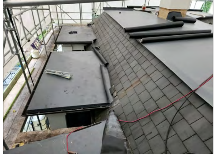
FLAGON TPO installation
