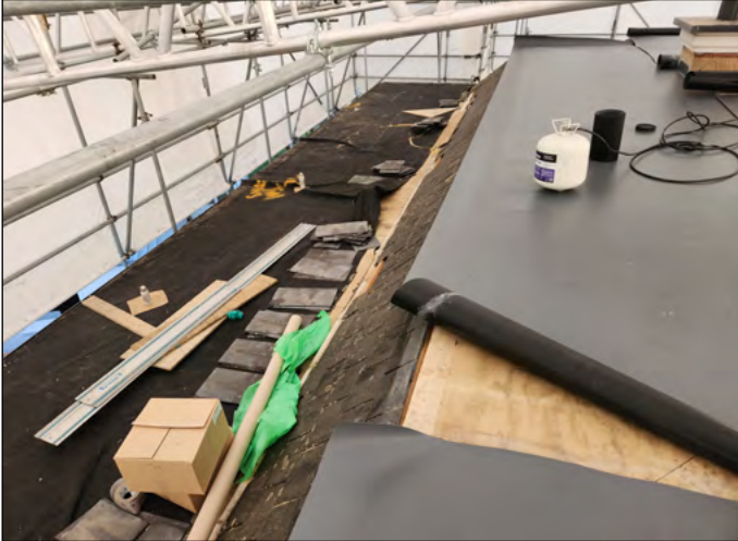
TPO Adhesive applied
