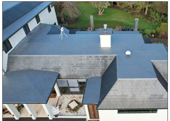
Finished portion of the roof in FLAGON TPO
