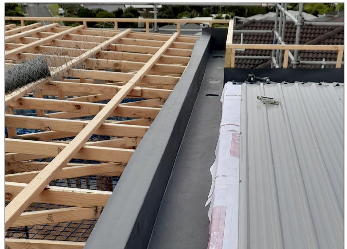
The FLAGON TPO membrane provides a smooth and aesthetical finish for internal gutters
