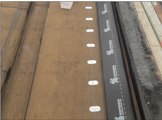
Base sheet in gutter area
