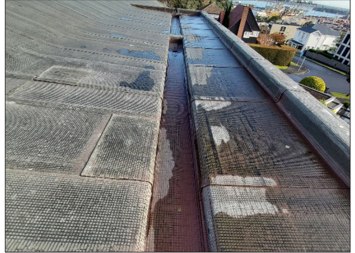
Existing membrane in gutters
