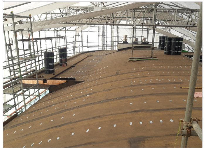
Base sheet mechanically fastened to existing membrane
