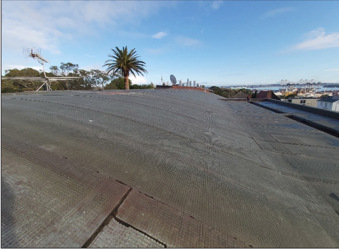
Existing copper membrane on curved roof
