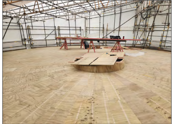
Installation of primer on plywood substrate
