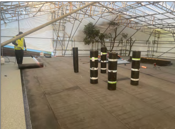
Installation of base- and cap sheet
