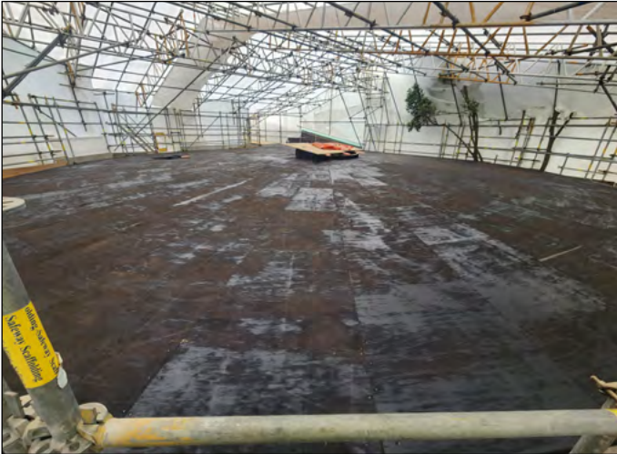
Installation of substrate
