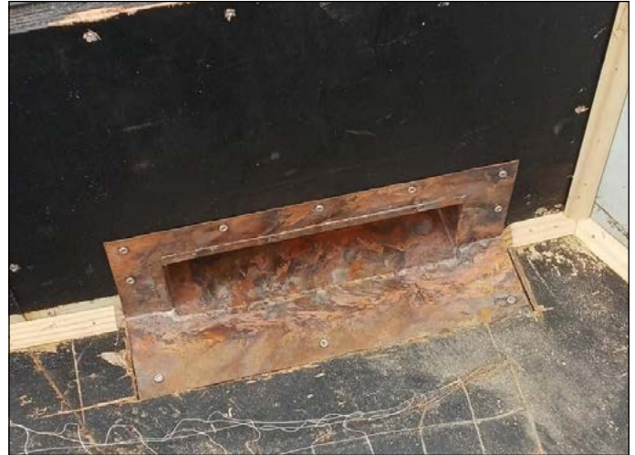
Installation of copper scupper drain
