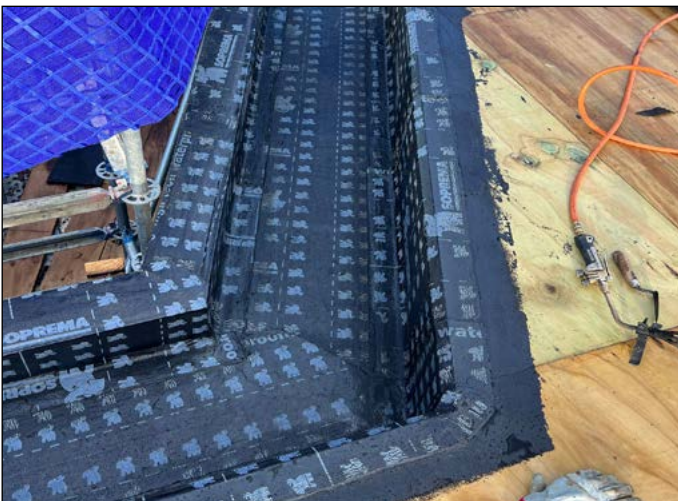
Installation of SOPRSUN PLUS 3 base sheet
