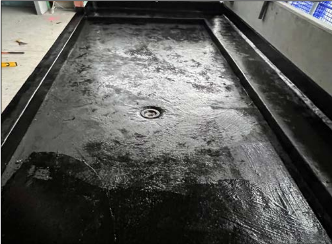
Application of SOPRADERE QUICK primer
