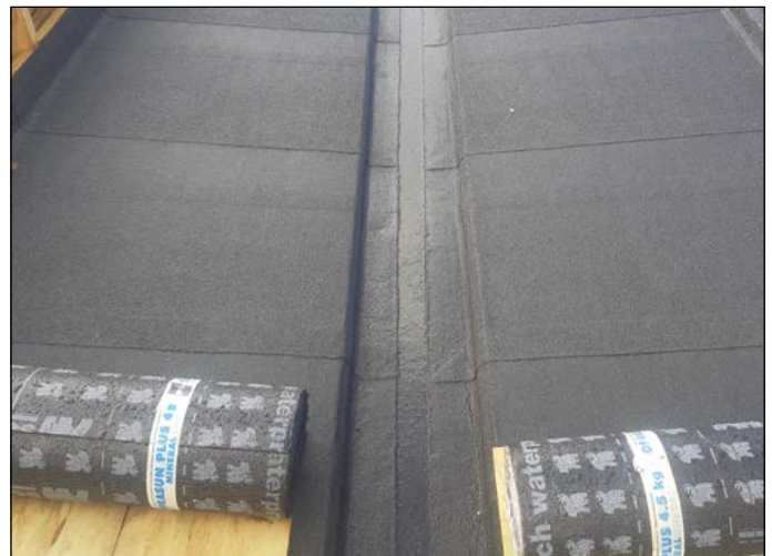
Installation of SOPRASUN PLUS MINERAL cap sheet
