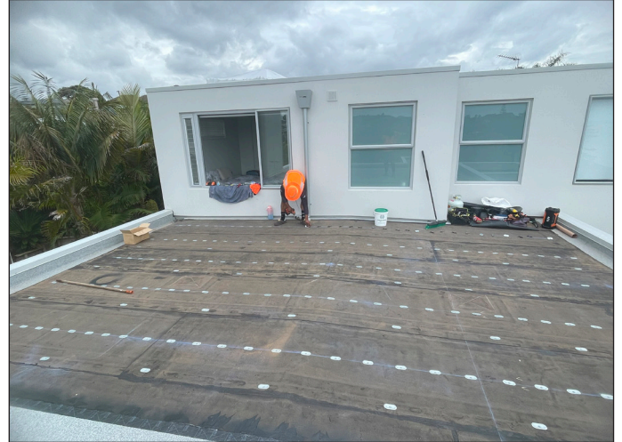
Base sheet mechanically fastened over existing membrane
