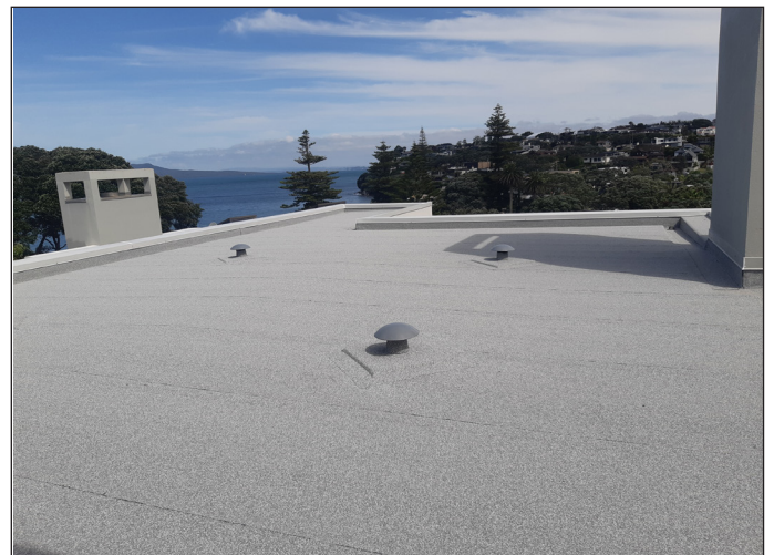
DUO cap sheet torched on over base sheet
