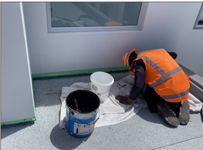
Under the cladding SOPREMA EASY FLASHING is used
