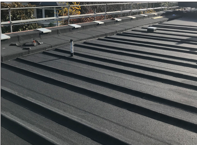
DUO cap sheet and solar panel plinths installed
