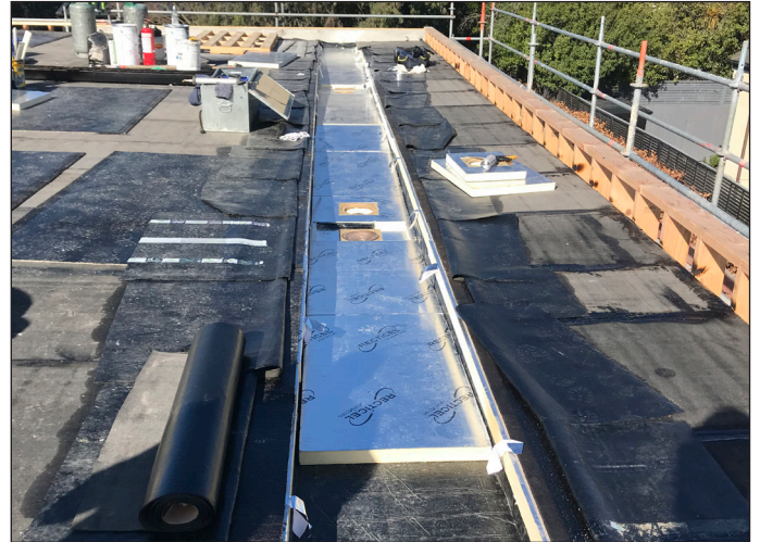
Thermal insulation installed under base sheet
