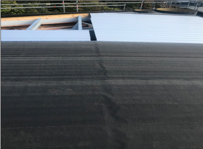
Debotack vapour barrier installed onto metal carrier tray
