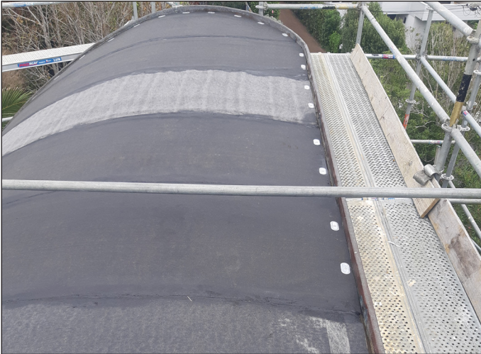
Base sheet mechanically fastened
