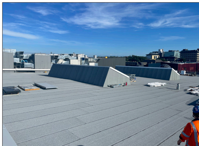
Detailing of DUO cap sheet
