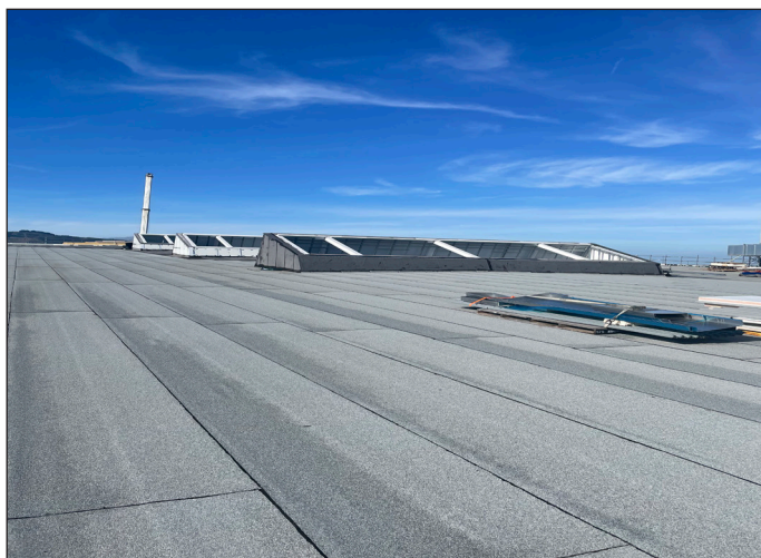
DUO cap sheet underway
