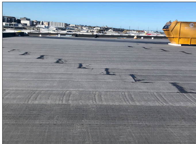
Debotack Aero base sheet being laid
