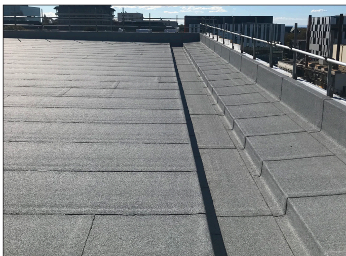
Completed DUOTHERM roof
