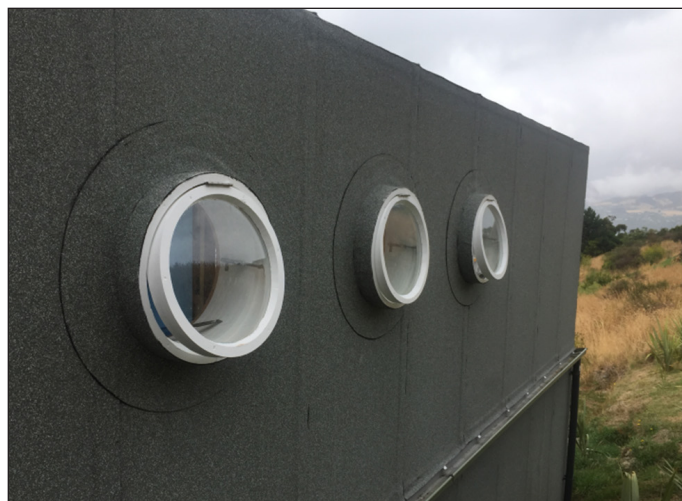
Completed detailing on windows
