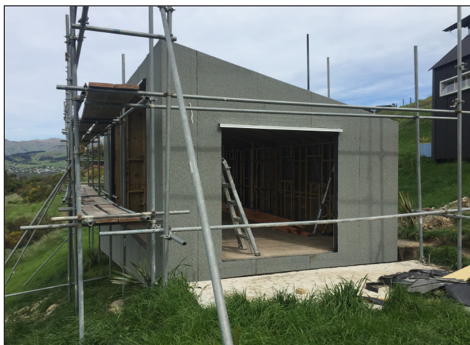
Finishing walls and detailing thresholds
