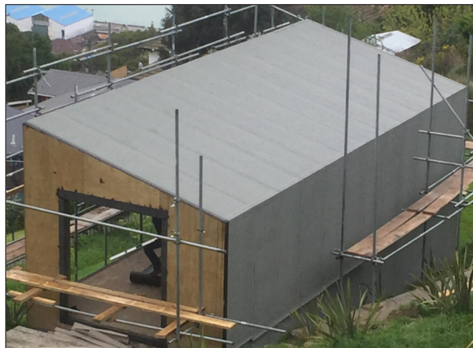
DUO cap sheet completed and connected on roof and back wall
