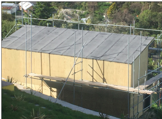
Deboflex base sheet being installed
