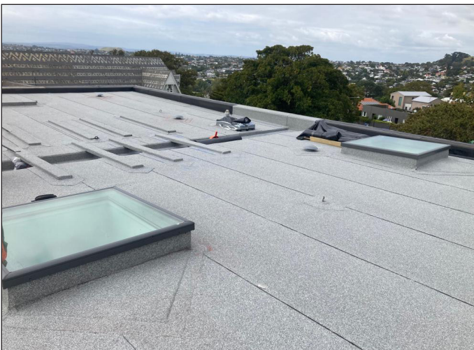
Membrane detailing to timber plinths with skylight cricket diverters completed
