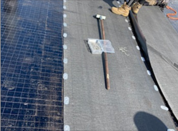
Mecano fixing plates with screws at 150mm spacings to mechanically fasten the Deboplast base sheet
