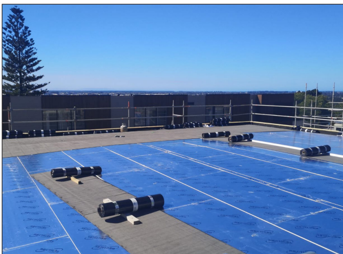
Installation of waterproofing base sheet
