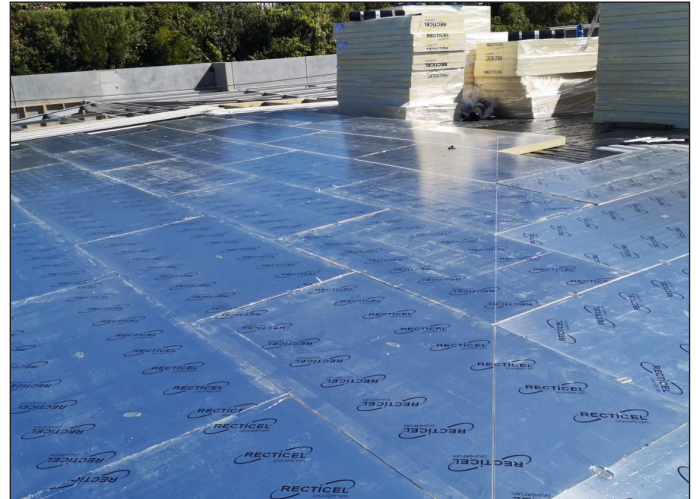
Installation of vapour barrier and thermal PIR insulation
