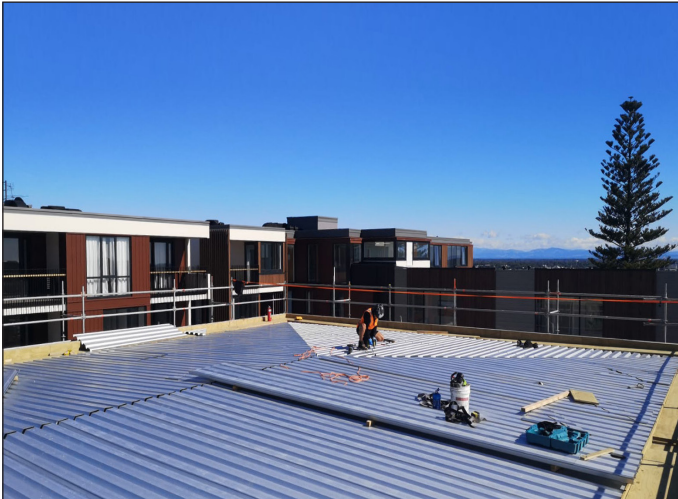
Metal substrate laid to fall
