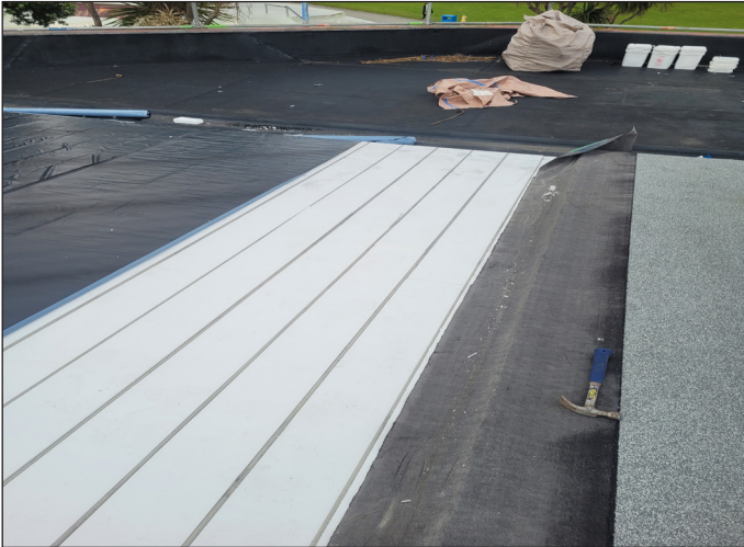
Vapour barrier over metal tray deck
