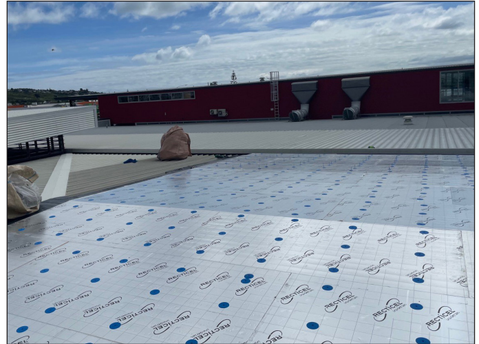
Installation of 81 mm Equus PIR insulation with Guardian fastening system
