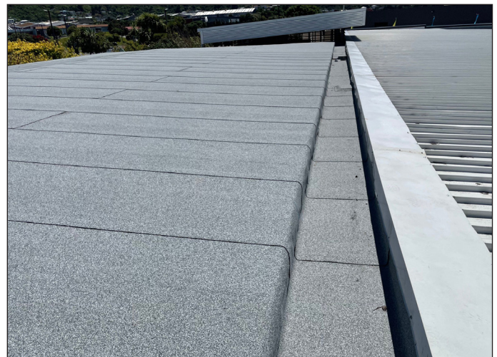
SOPREMA DUO cap sheet (GW) installation
