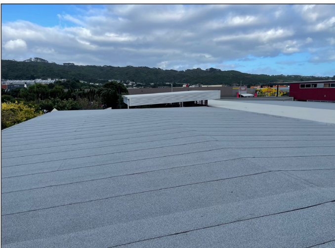
Completed DUOTHERM Warm Roof
