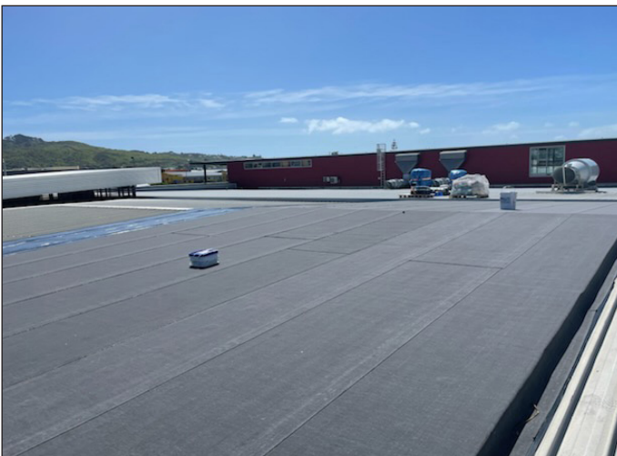
SOPREMA Debotack Aero base sheet Installation
