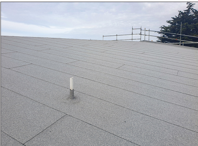
Completed DUO membrane installation
