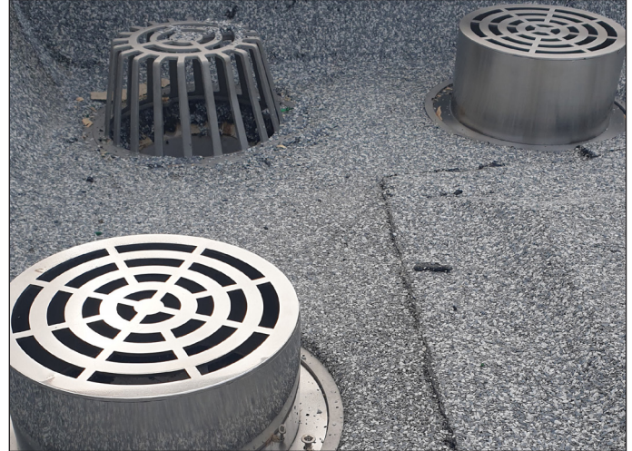
Installation of DUO membrane showing detailing
