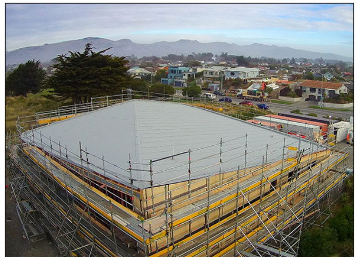
Completed DUOTHERM warm roof
