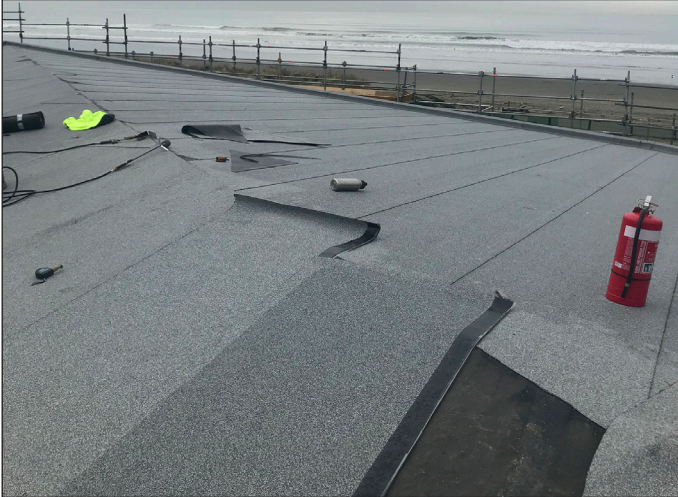
Installation of DUO cap sheet
