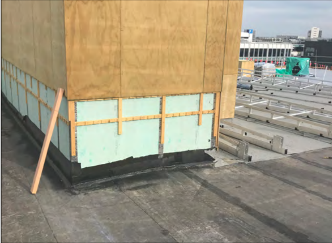
Installation of DUO base sheet
