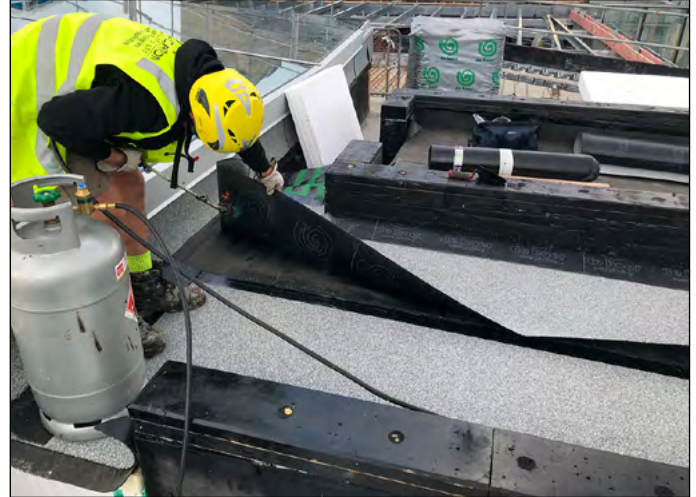
Installation of DUO cap sheet
