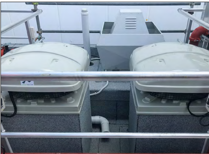
Installation of DUO membrane to details
