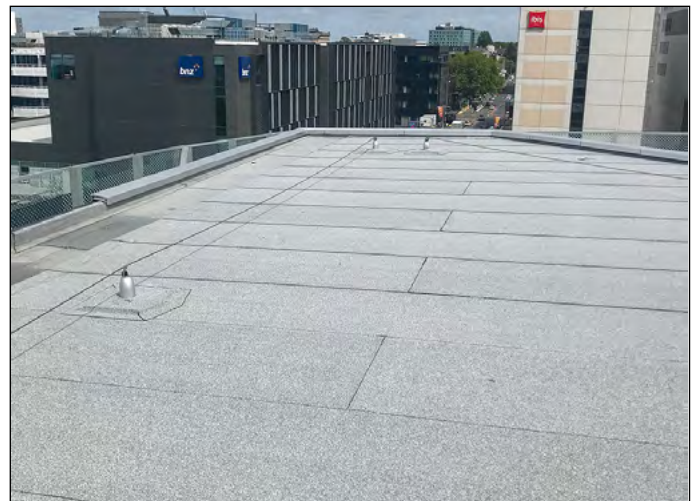
Completed DUOTHERM warm roof
