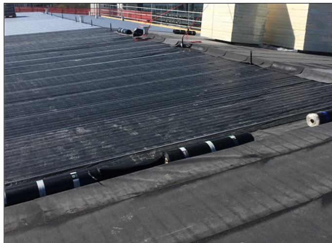
Base sheet application over PIR thermal insulation board
