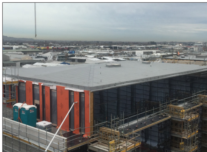
Completed DUOTHERM roof
