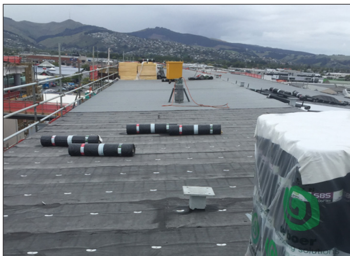
DUO capsheet application over base sheet
