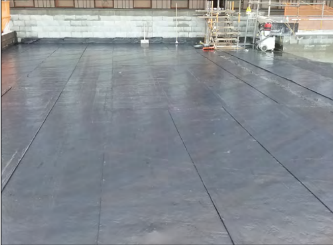
Vapour barrier installed
