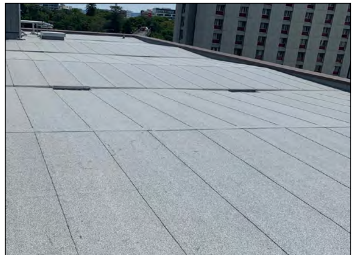
Finished cap sheet
