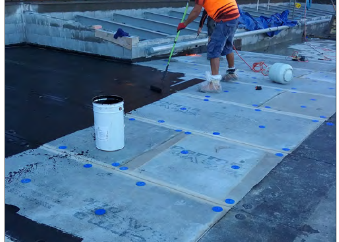
Permabase Dek installed with mechanically fastened ASTL plugs and then primed
