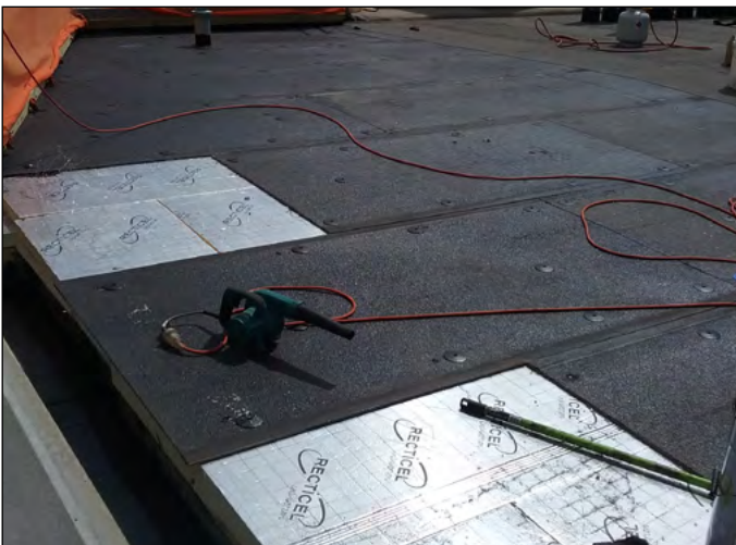
PIR installed with primed Permabase Dek
