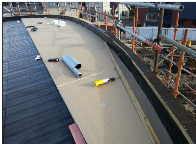
Installation of PIR Board over vapour barrier
