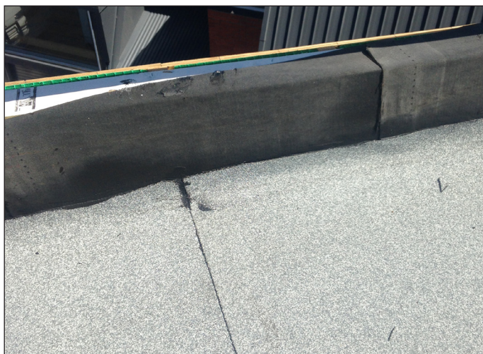
Soprema DUO cap sheet application
