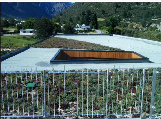
Finished project—mixed use roof concept
