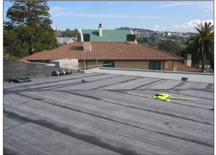
DUO base sheet installed to the roof
