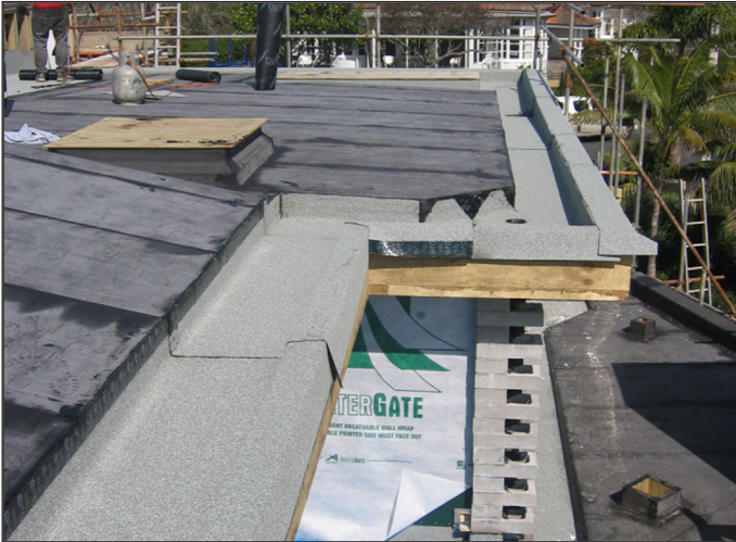
DUO base sheet & cap sheet installed to the gutters
