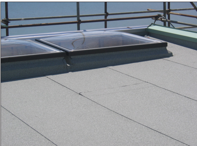
DUO cap sheet installed to the roof
