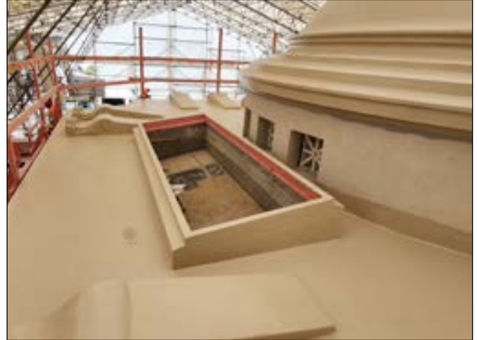
Chevaline Dexx bodycoat application in progress on dome and platform base
