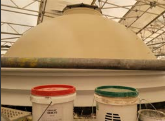
Dome refurbishment in progress with Chevaline Dexx bodycoat application
