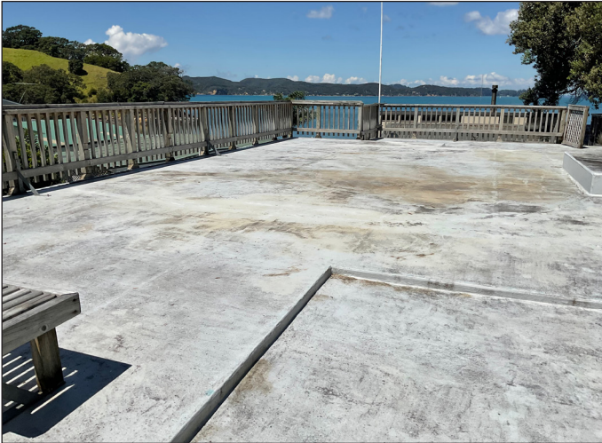
Original garage roof/deck
