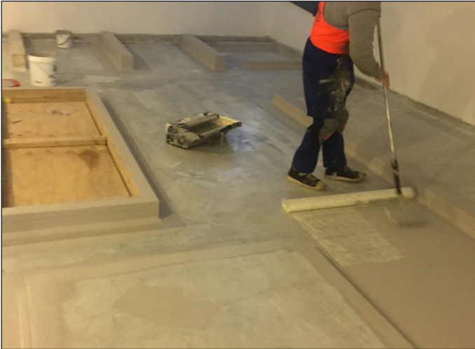
Fibreglass reinforcement laid into wet Chevaline Dexx bodycoat
