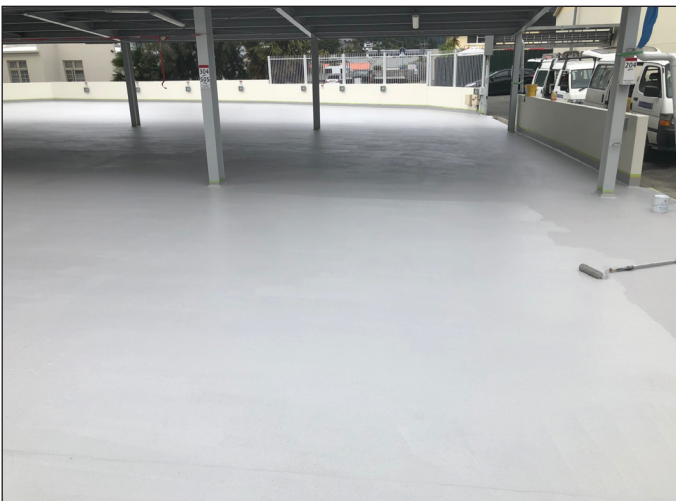
Traxx Topcoat application over finished Dexx Membrane
