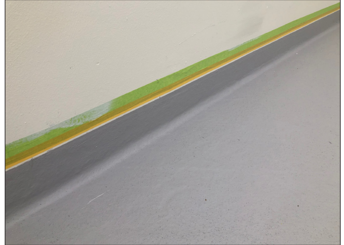
Chevaline Dexx Membrane applied to upstands
