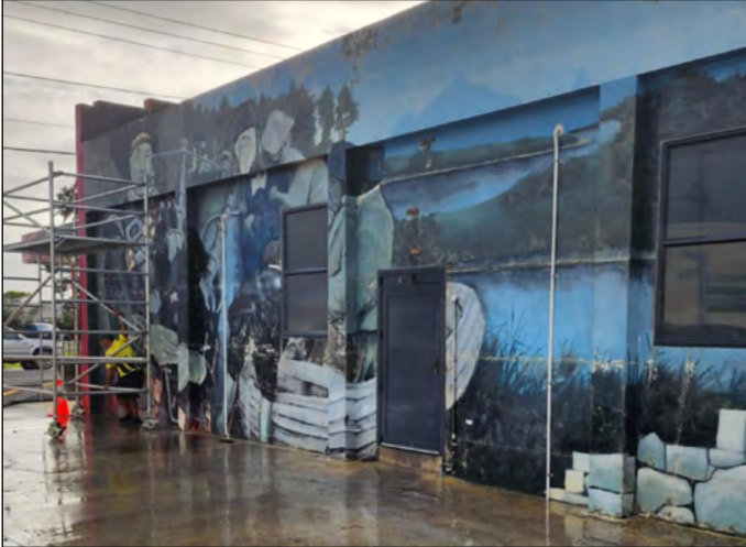
Preparation for cleaning building
