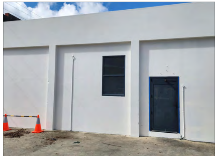
Chevaline Coverflexx NF bodycoat applied
