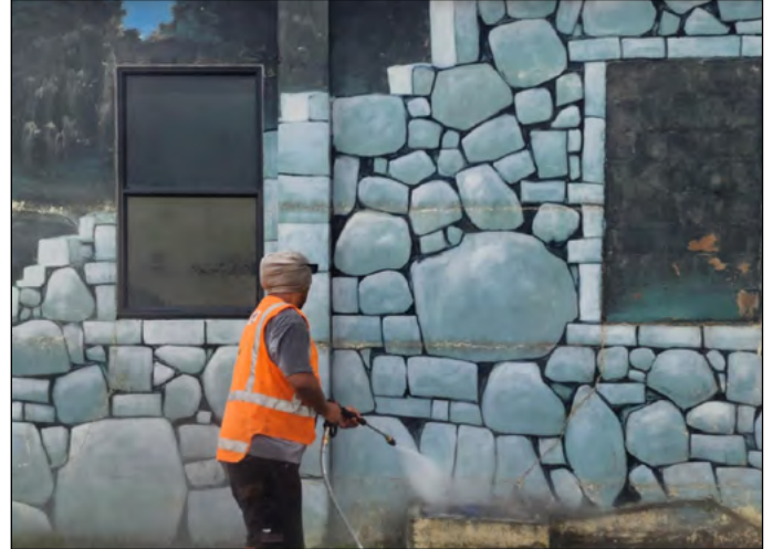
Mosskill and waterblasting of building
