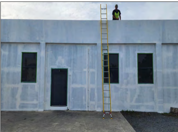
Repairs completed and Epistix primer applied
