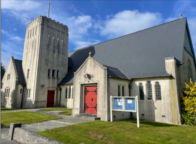
Before preparation has started
