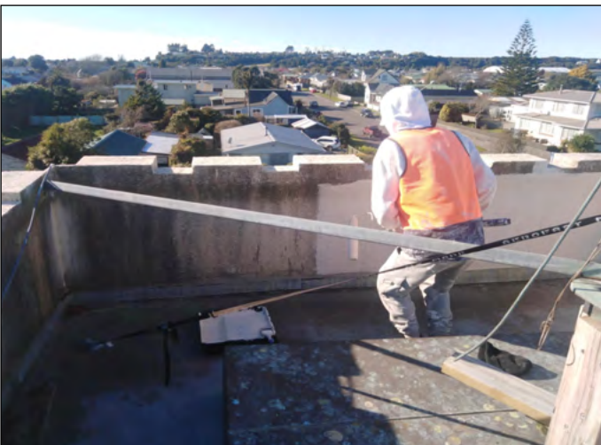
Application of Keim Granital Grob basecoat
