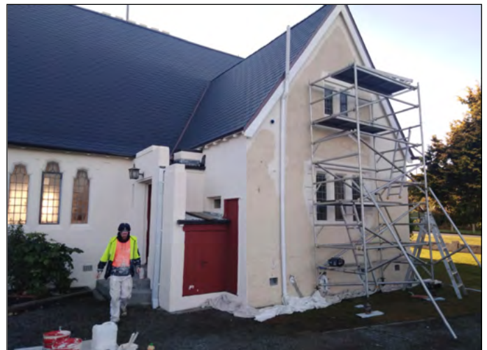
Final coat of Keim Granital topcoat being applied
