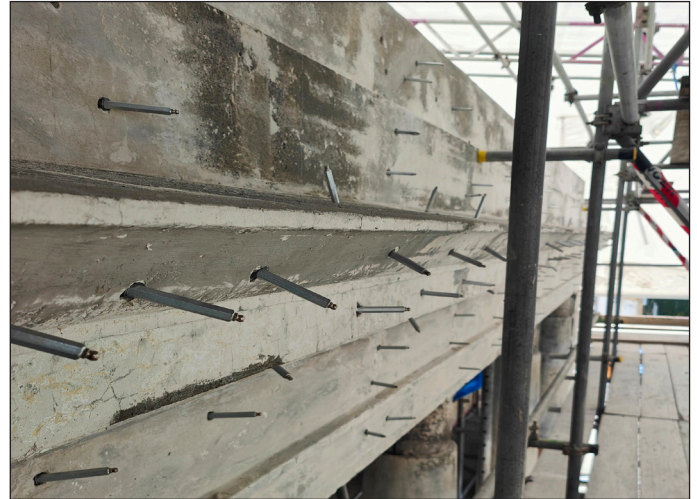
Crack injection before paint application
