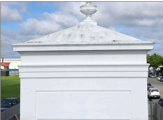
Primed with Chevaprime-U and Coverflexx application
