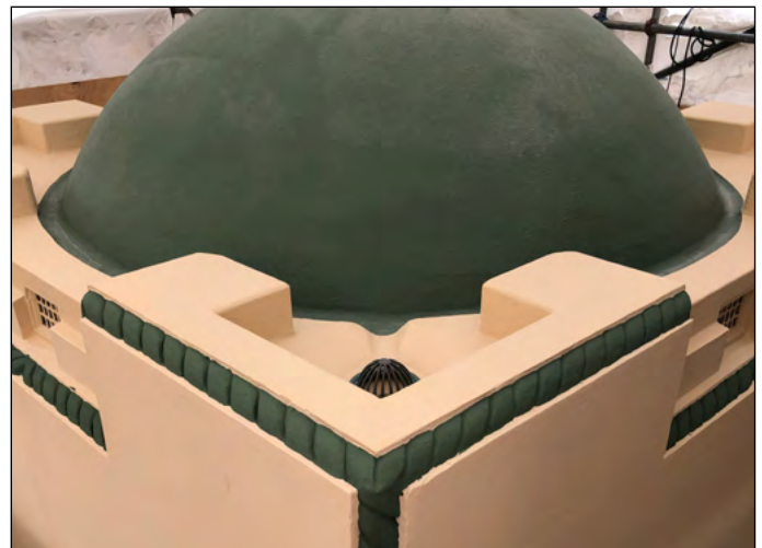
Chevaline Dexx application to dome roof and drain areas
