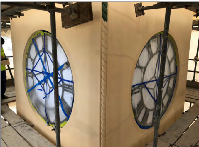
Crack repair and Keim Granital application to clock tower walls
