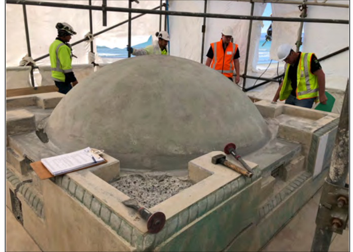
Preparation for Chevaline Dexx application to dome roof
