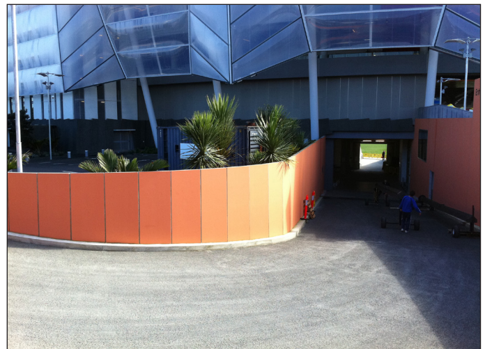
Finished Keim coatings to entrance barriers
