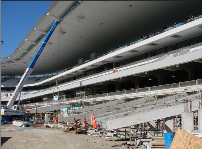
Construction of South Stand
