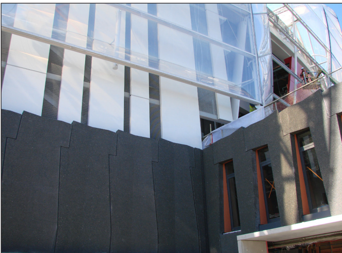
Finished Keim coatings applied to concrete
