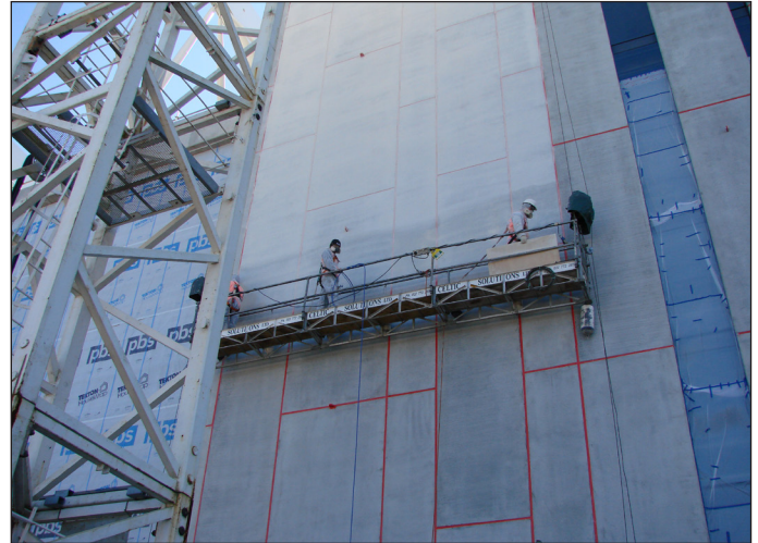
Keim Concretal Lasur coating application to concrete panels
