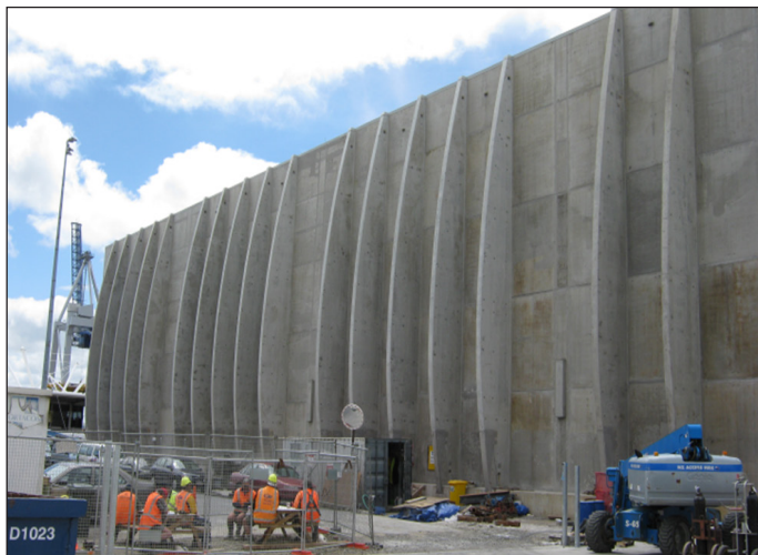
Substrate prior to cleaning and preparation
