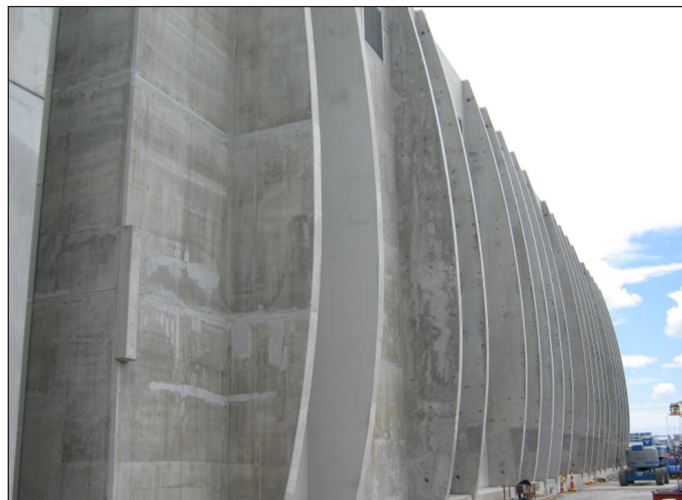
Trial fin completed
