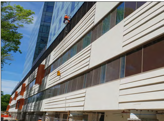
Keim Granital application on concrete panels
