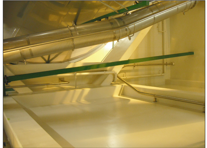
Chevaline Colourglaze to interior concrete
