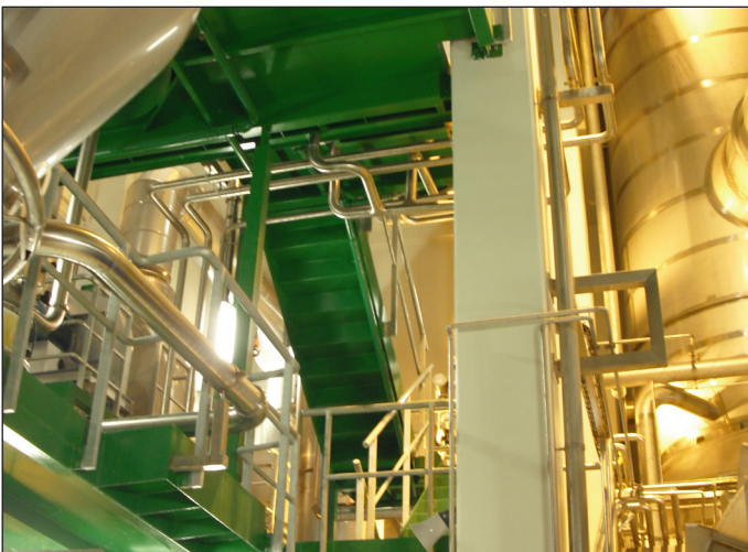
Colourcure to steelwork
